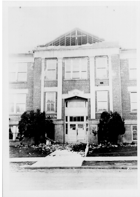
1949 earthquake, Washington State. Gables on a number of unreinforced masonry school buildings collapsed; fatalities recorded
